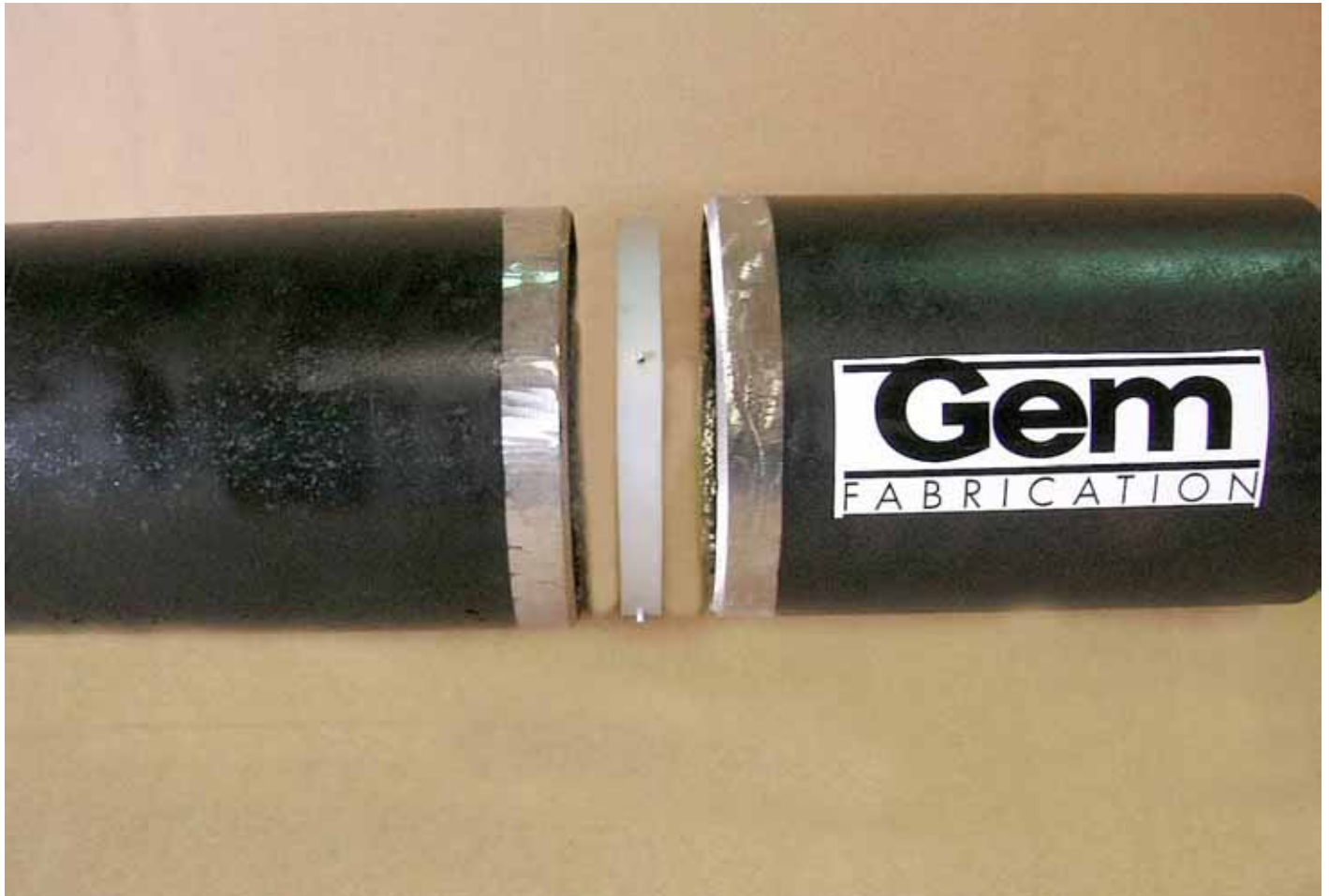
Pipe and backing ring shown prior to installation
